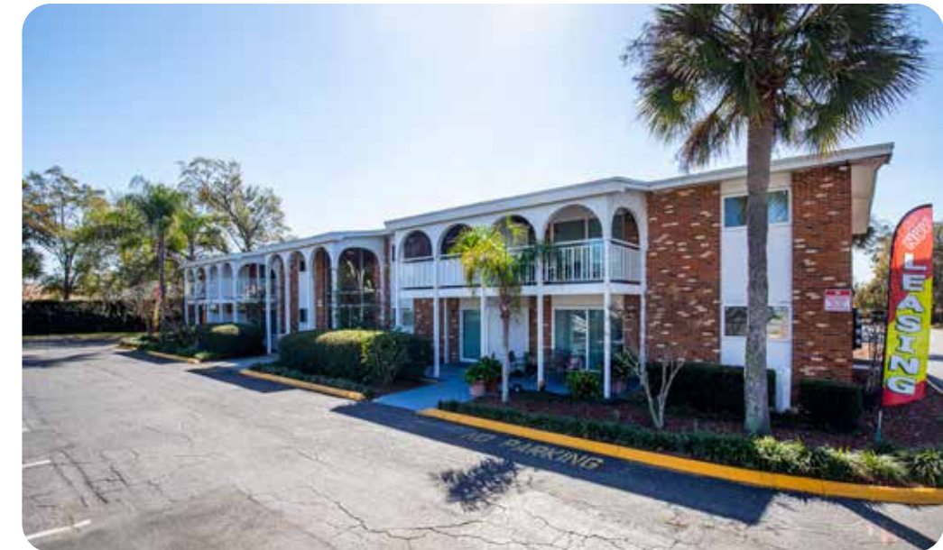
Install key fob access on interior corridor building
